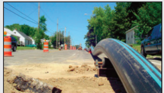
12" HDPE going into a pipe burst in Ft. Wayne last year.
