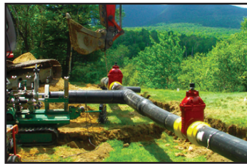
HDPE main line with inline butt fusible AVK valves installed.
